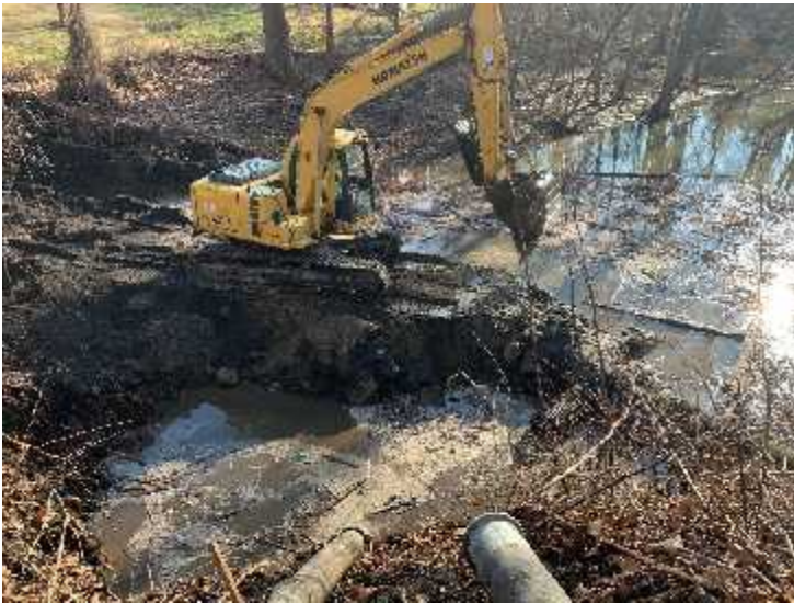
Construction Cofferdam
