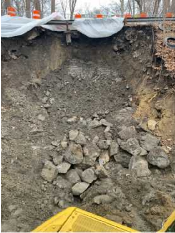
Insertion of Steel Sleeve Pipe
